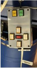
To close the upper shutter, ensure the lower slot door is closed. Rotate the dome until the slot motor assembly is located above dome bearing assembly '1'. Using the 'CLOSE' button on the hand pad, close the upper shutter. The limit switch will operate when the shutter is fully closed.
