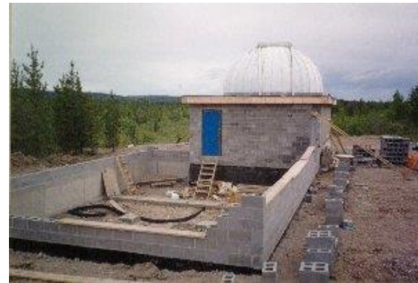
Above: Construction of the Classroom on May 1993
