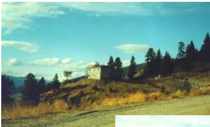
Jack Newtons B&B under construction on Anarchist mountain.
