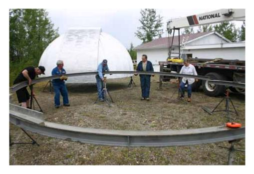
The ring halves were set on adjustable jack stands donated for the day by Central Interior Piping for the trimming and welding into one seamless circular beam. Sterling Crane's Tom Volk lifted off the dome.
