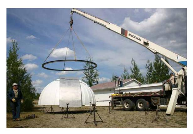
Once the ring beam joined we test rotated it on the rollers and it fit perfectly. Once the ring beam was confirmed to fit and rotate freely on the rollers, the beam was then painted, since some parts would not be accessible later.
